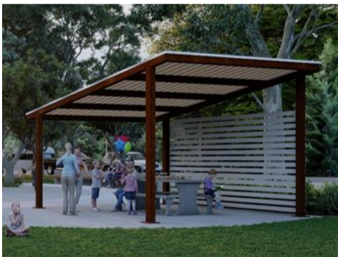
COLORBOND SKILLION ROOF TO POWDER COATED ALUMINIUM STRUCTURE. OVERALL STRUCTURE SIZE 5700x4600mm. WHITE HORIZONTAL SLAT TO 2450mm HIGH TO 3 SIDES OF STRUCTURE.
