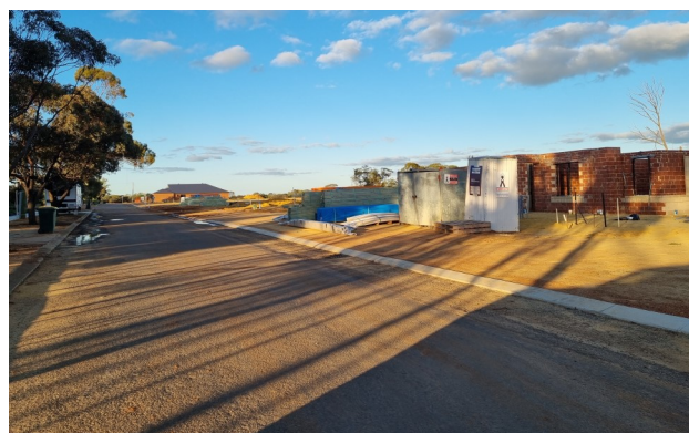
Bell Street Subdivision June 2021
